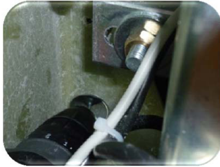
Picture 5: Loosen and remove all fastening screws (left and right).
