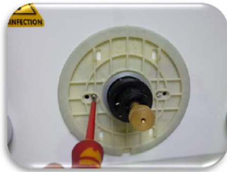
Picture 9: Loosen and remove the left and right screws from the thermostat mounting plate.
