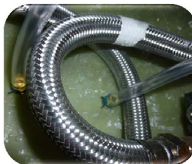
Picture 4: The illustration shows the flow meter in installed condition.
