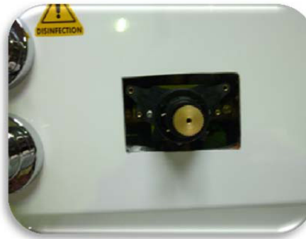
Picture 10: The illustration shows the exposed thermostat. Now the inserts (filter, etc.) can be taken out and replaced.
