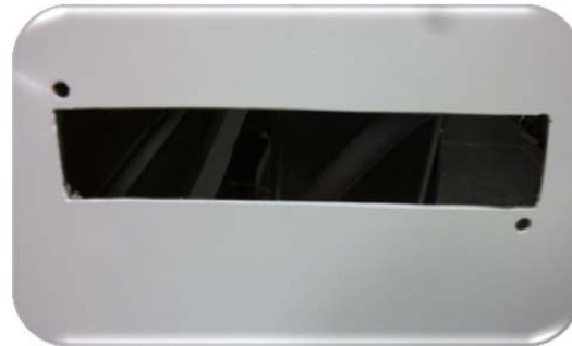
Picture 10: The illustration shows the recess in which the operating element is installed.
