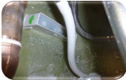
Picture 7: The illustration shows the operating element with threaded connection loosened (inside view).
