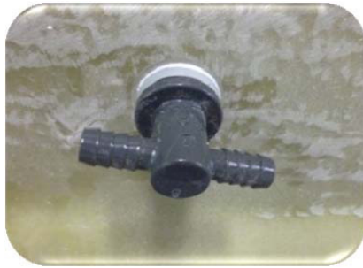
Picture 13: Loosen and remove the connecting valves by turning in counter-clockwise direction.
