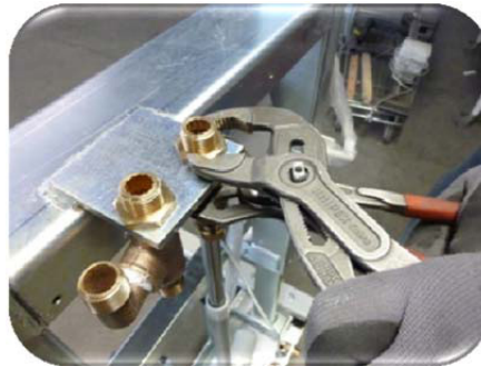
Picture 16: Loosen the nuts for the hot water connection using the two pipe wrenches.
