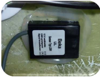
Picture 7: Affix the new sensor at the old position.
