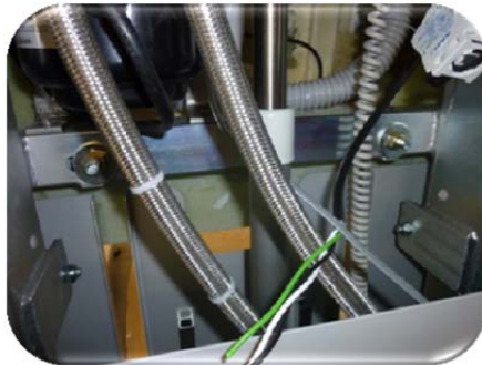
Picture 9: The illustration shows the lower fastening screws.
