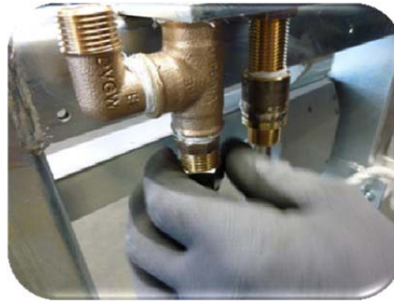
Picture 14: Remove the union nut from the thread of the connection for cold water.
