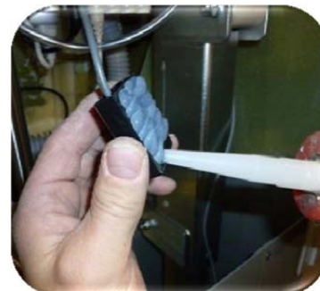
Picture 6: Apply a layer of transparent silicone to the reverse side of the sensor and place it at the position of the old sensor.
