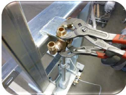
Picture 15: Loosen the nuts for the cold water connection using the two pipe wrenches.
