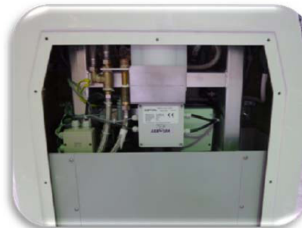
Picture 2: The illustration shows the disinfectant container installed in the control panel.
